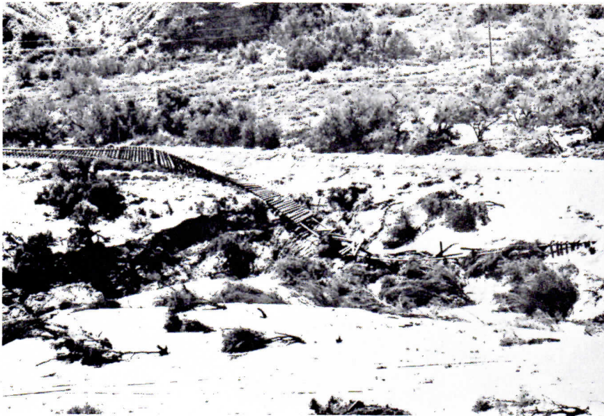
Figure 5. Railroad damage in Moapa Valley.
